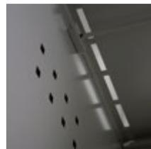
Ventilation in the shelf – air flows from the floor through vents in the shelf to the vents above the door.
